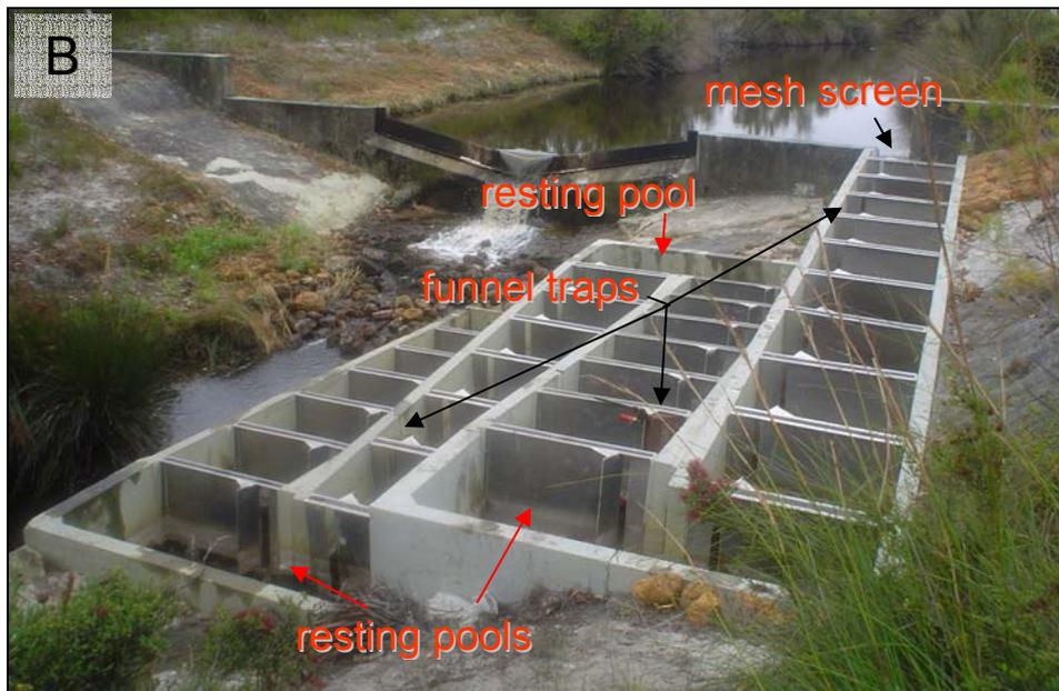
Plate 2 (A) Mesh screen and funnel trap set on the Goodga River Fishway during each sampling occasion and, (B) the location of the funnel traps, mesh screen and resting pools on the fishway.
