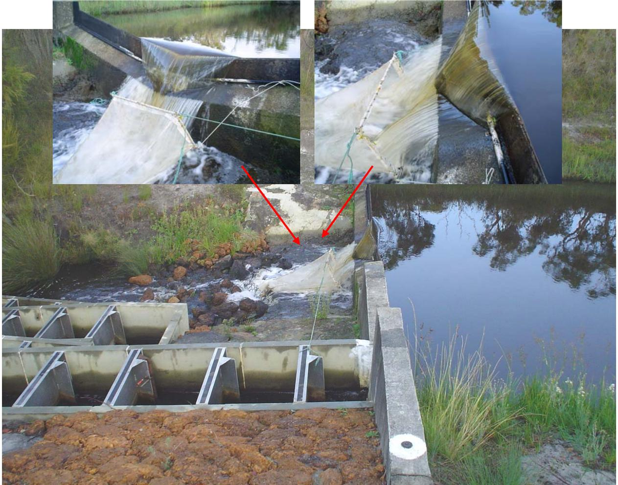
Plankton net set below the Goodga River Gauging Station to determine the extent to which fish moved downstream over the wall.
